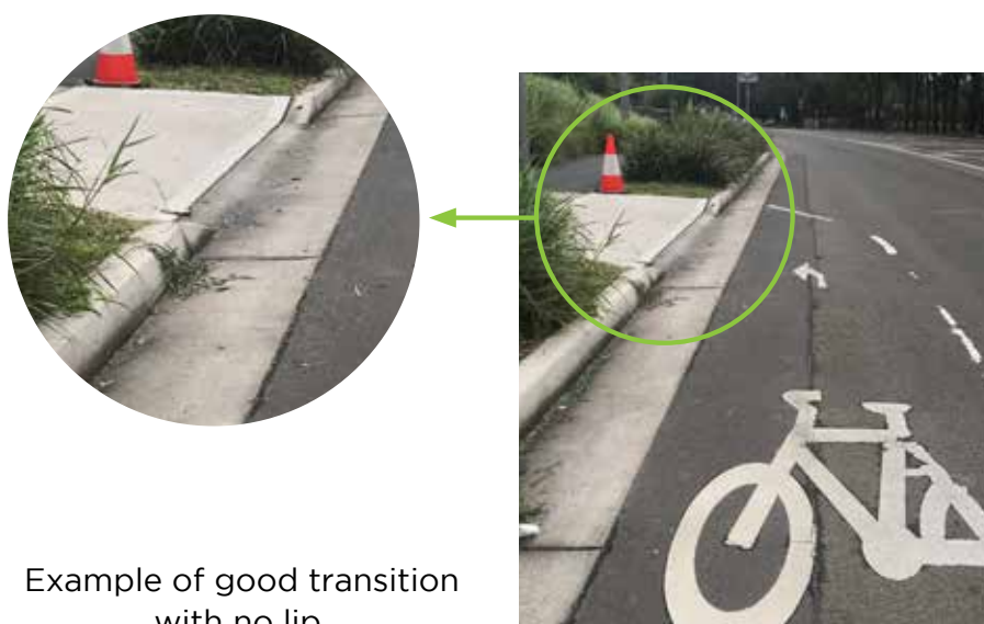
Figure 8.6: An example of a kerb ramp design
