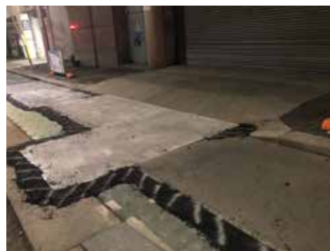
Smooth road-plates with a non-slip surface, hotmix used for smooth transition and clearly marked edges.
