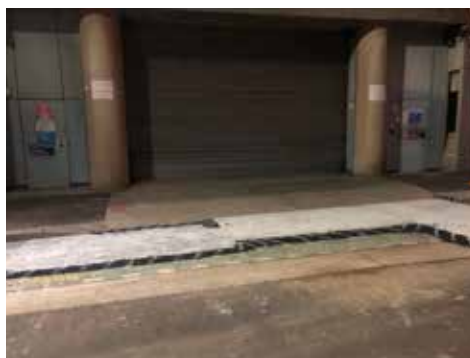
Smooth road-plates with a non-slip surface, hotmix used for smooth transition and clearly marked edges.
