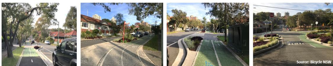
Figure 6: Bi-directional separated cycle paths on Sutherland Street and Young St in the North Sydney LGA. The paths are raised to pavement level and protected from vehicle traffic by a parking and landscape buffer.
