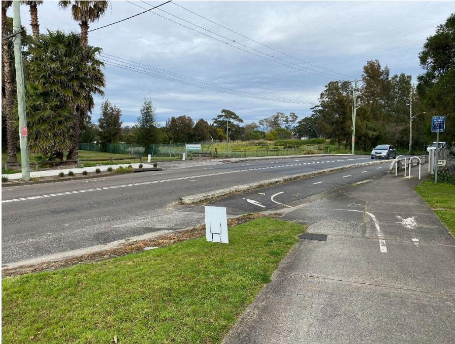
Figure 4: Bestic Street is a major junction point of the future regional cycleway corridor and is currently non-compliant for bicycle use. Bicycle NSW seek a safety upgrade of this crossing.
