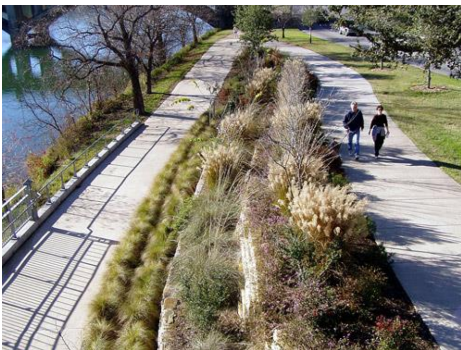
Figure 4: Separate paths for walking and cycling reduce conflict and minimise the visual and environmental impact of widened shared paths (Source: http://www.pedbikeimages.org/ - Dan Burden)
