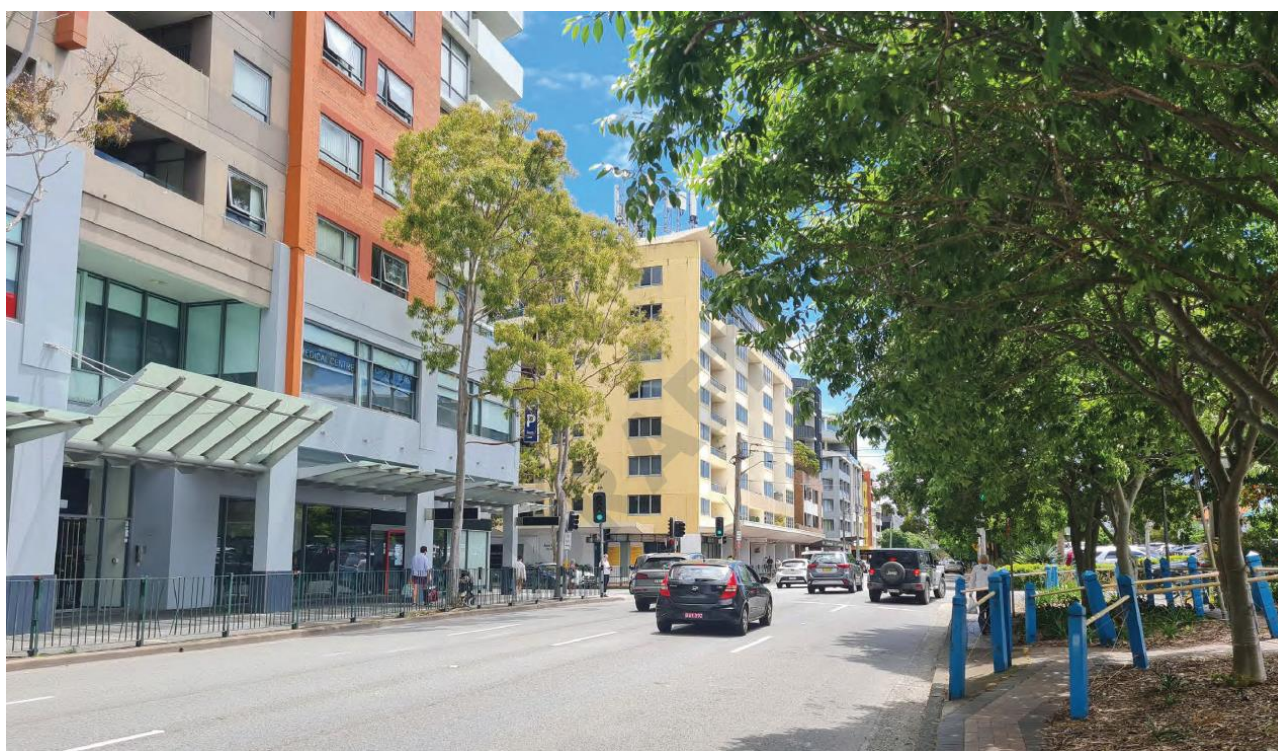
Figure 1: Anzac Parade, Maroubra Junction - a multi-lane road slices through the commercial centre, pedestrians are penned into narrow footpaths by fencing so cars can pass unimpeded at dangerous speeds, pedestrian realm is poor and unwelcoming, and there are limited opportunities to cross the road. (Source: Randwick City Council)
