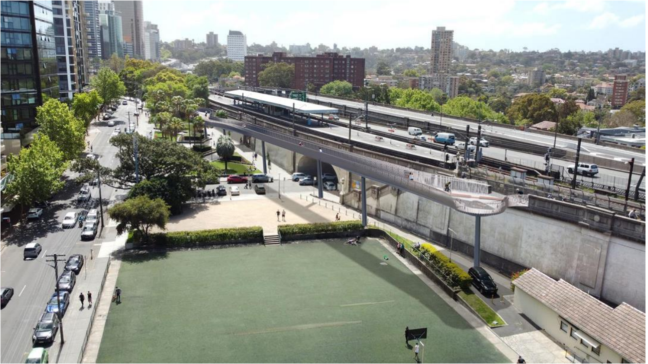
The award winning linear access ramp complements the heritage of the SHB profile and Bradfield Park. ( Aspect Studios )
