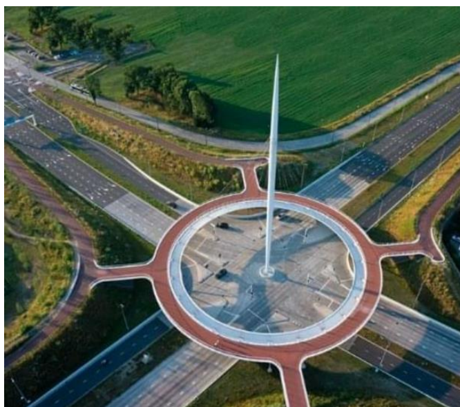
Figure 9: The Hovenring provides safe, seamless and transformational active transport connections across a major road junction in Eindhoven, the Netherlands. It is a landmark structure that touches the ground lightly and celebrates walking and cycling (Source: https://hovenring.com/ )
