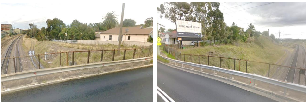
Figure 3: Looking down into the rail corridor from the Maud Street bridge, to the south (left) and north (right). It is clear that there is a wide easement. Minimal stabilisation would be required for a 3-4m wide shared path (Source: Google Maps)
