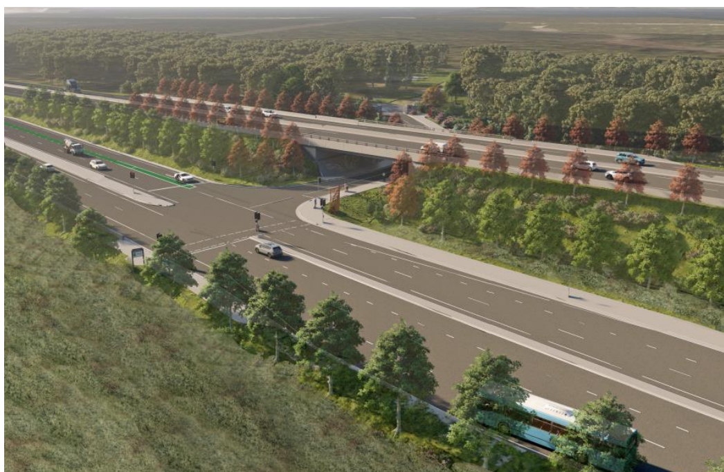
Figure 4: Aerial View Black Hill Interchange looking East showing enhancing shared path and active transport connections from HRBG to Pacific Highway.
