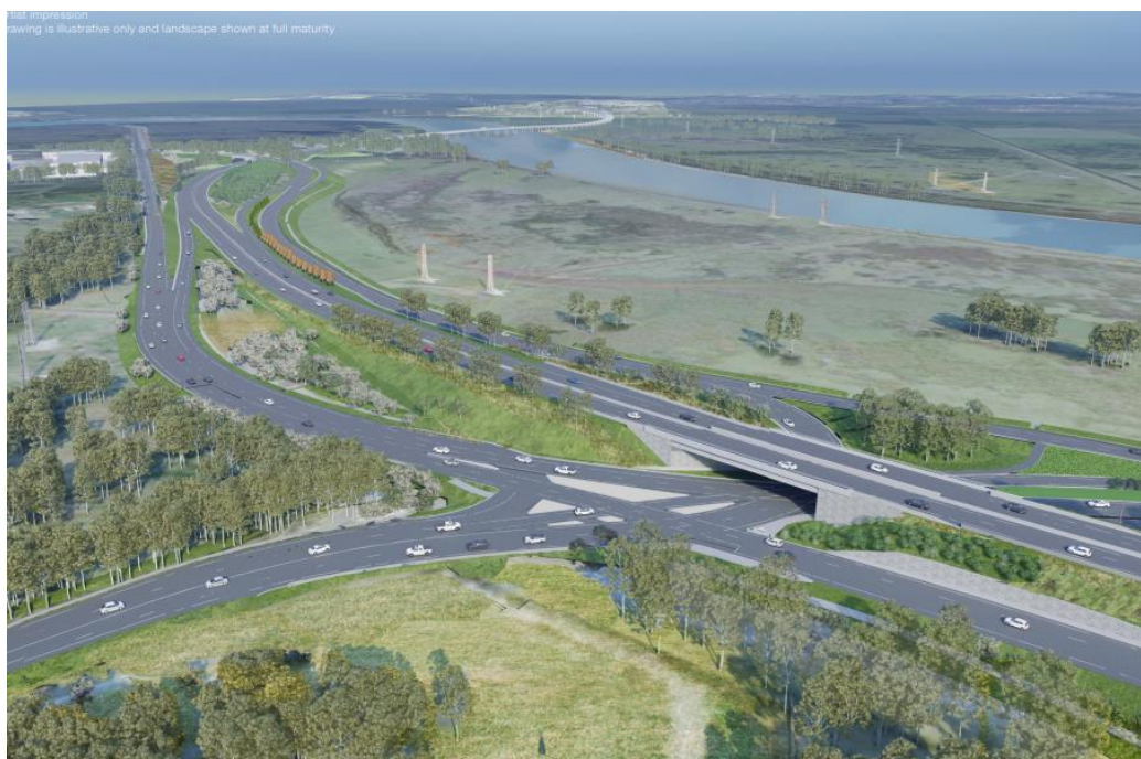
Figure 3: Aerial View Tomago Interchange looking West
