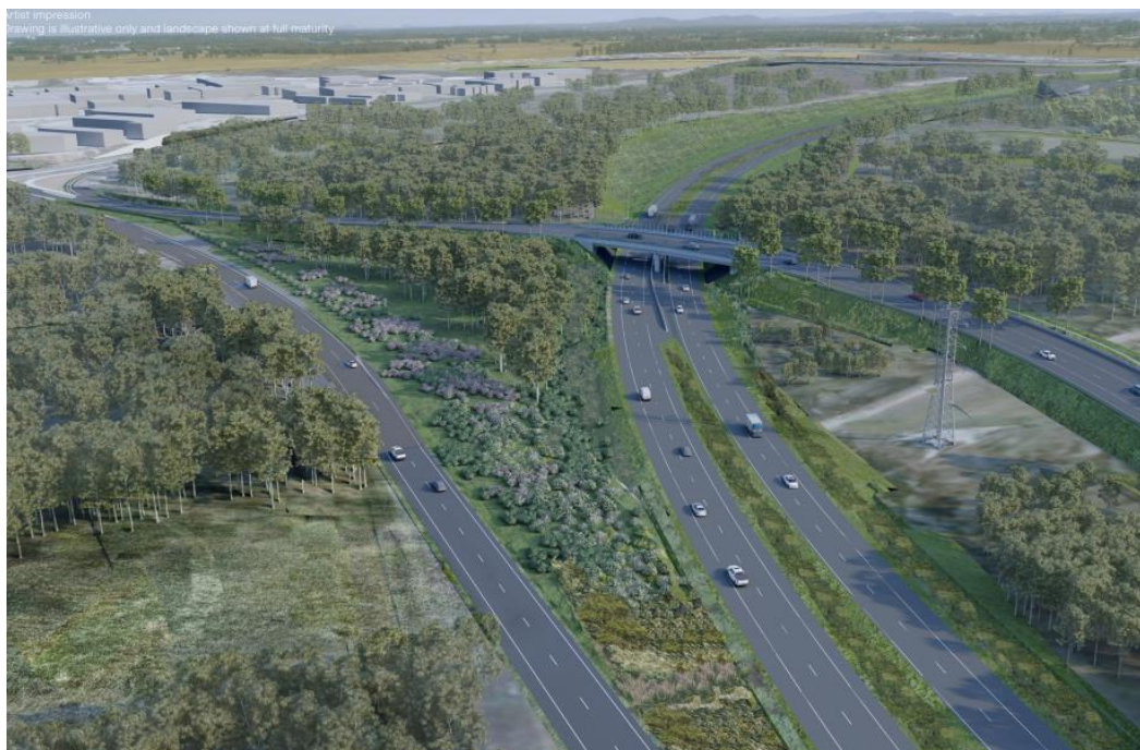
Figure 2: Aerial View, Black Hill Interchange looking North.
