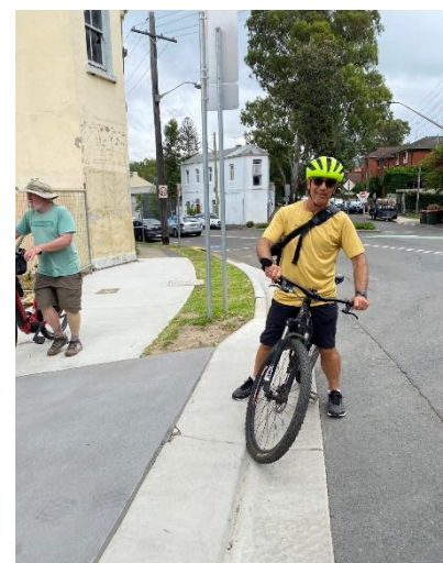
Figure 5: An Inner West Bicycle Coalition advocate show where a 5cm high lip has been incorporated into a dropped kerb – on a cycle route! (Image: Bicycle NSW)
