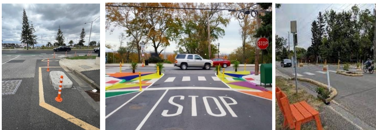
Figure 5: Bolt-down concrete pads, posts and paint create simple kerb extensions to slow cars turning from Marine Parade, St Kilda (left, image: Bicycle NSW) Painted kerb extensions make streets safer by shortening the crossing distance for pedestrians and improving visibility for turning cars (centre, image: Brian David Platt ). Thick coir rope can be used to form chicanes and blister islands (right, image: Bike Walk Montana )
